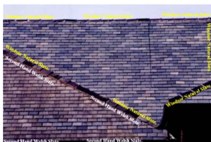
Reclaimed Welsh Slate on the same Building.
